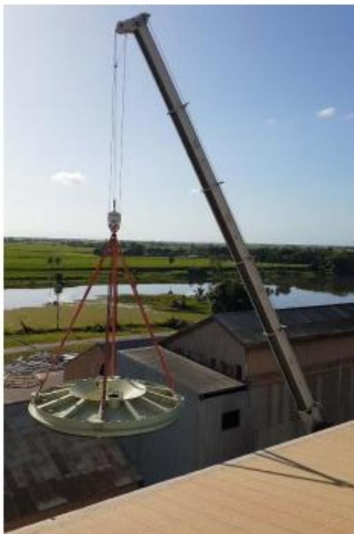
A crane is used to lift the bottom cone section of the new Kalamia Mill evaporator into the factory.
