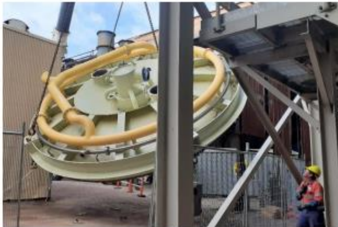
Rigger Pete Daley directs the flip for the bottom cone of the new evaporator at Kalamia Mill.
