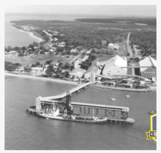
Pictured: The Lucinda sugar terminal located approximately 100km north of Townsville. The jetty seen here was constructed in 1958 and runs to a length of 210 metres. However, to accommodate larger ships used in the bulk raw sugar trade, in 1979 a new jetty was built which stretches nearly 6km out into Halifax Bay and is the longest service jetty in the Southern Hemisphere.
