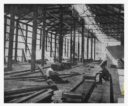
Pictured: Construction of the new sugar storage shed in Carins ca 1923. Located in the Cairns Wharf Complex, this heritage-listed sugar storage shed (known as White's Shed) played a crucial role in handling sugar bags for transportation. An electrical conveyor system was installed in the shed to move sugar bags to and from shipholds and railway wagons in 1926. Photo courtesy of State Library of Queensland.
